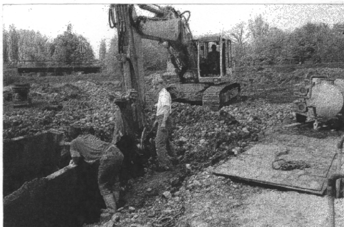
Excavation of the Henrichenburg Castle
