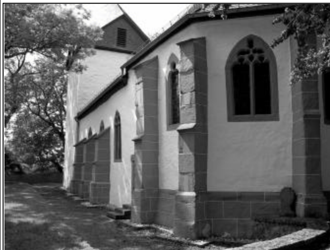
The Old Catholic Church at Alendorf, Germany. The church had just been freshly painted in 2004.
