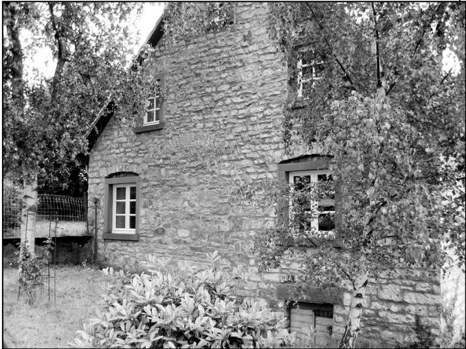
Side view of the original Heck family home at Alendorf, Germany in 2007.
